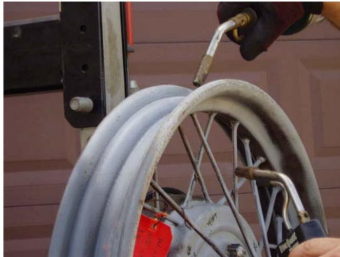
HEAT THE BASE OF THE SPOKE YOU HAVE CHOSEN TO SHRINK FROM THE TIRE SIDE OF THE WHEEL AND ALONG THE ENTIRE LENGTH OF THE SPOKE AT THE SAME TIME.
