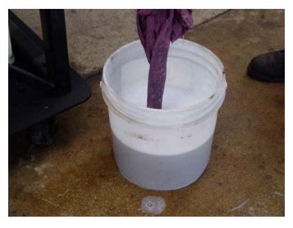
I USE A SOAPY MIXTURE OF COLD WATER TO COOL THE SPOKES. AN OLD SECTION OF A COTTON TOWEL WORKS WELL TO HOLD A LOT OF WATER.
